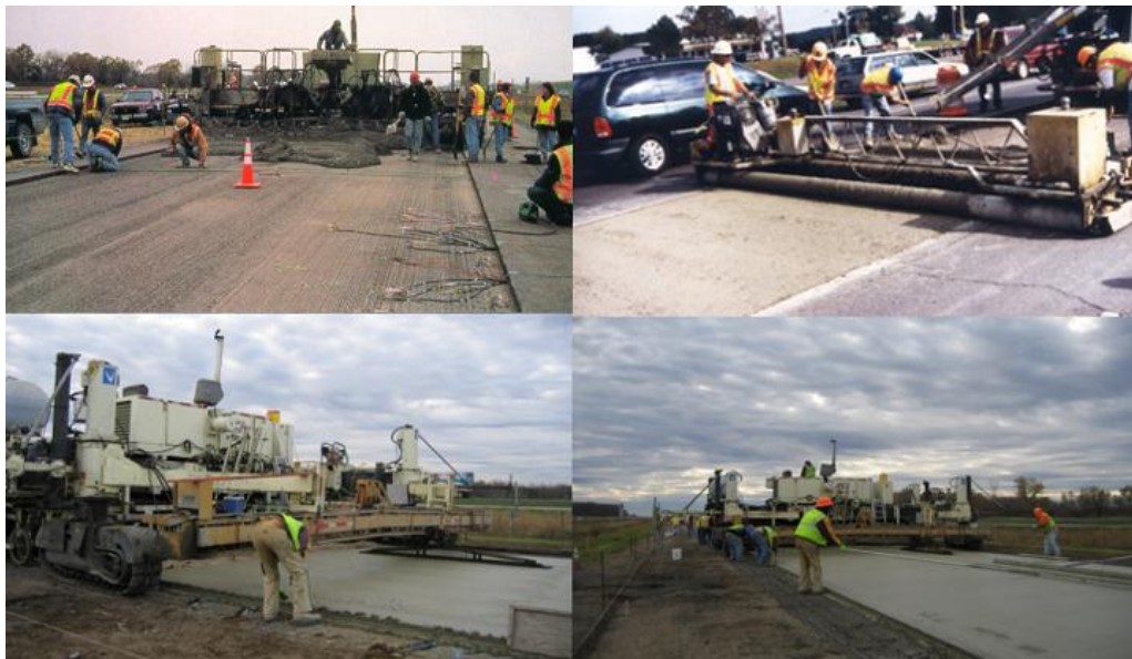
Figure 10. Placing and finishing the mill and fill BCOA.
