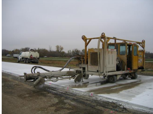
Figure 11. Sawing joints
