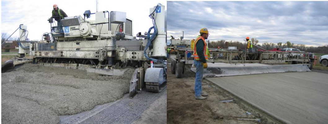
Figure 14. Paving and finishing an unbonded overlay
