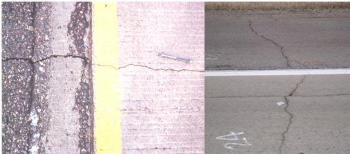
Figure 2. Reflective cracking in a BCOA
