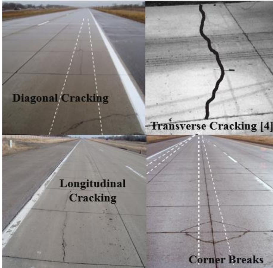
Figure 1. BCOA load-related distresses.
