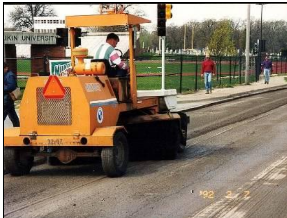
Figure 9. Sweeping the HMA surface after milling.
