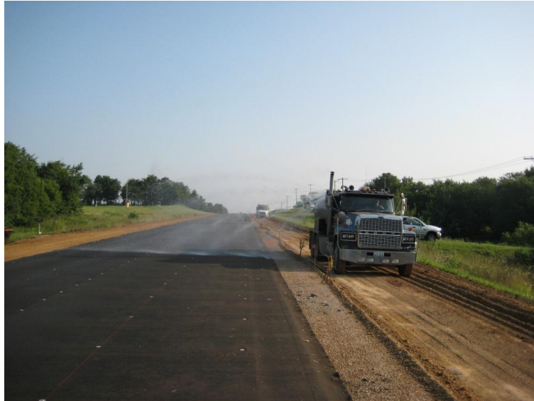
Figure 13. Misting interlayer prior to paving the unbonded overlay. (Photo courtesy of John Donahue of the Missouri Department of Transportation.)
